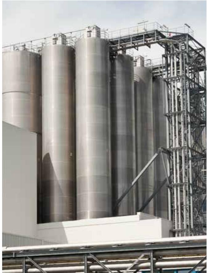
**Figure 10** Storage of precipitated silica in silos
